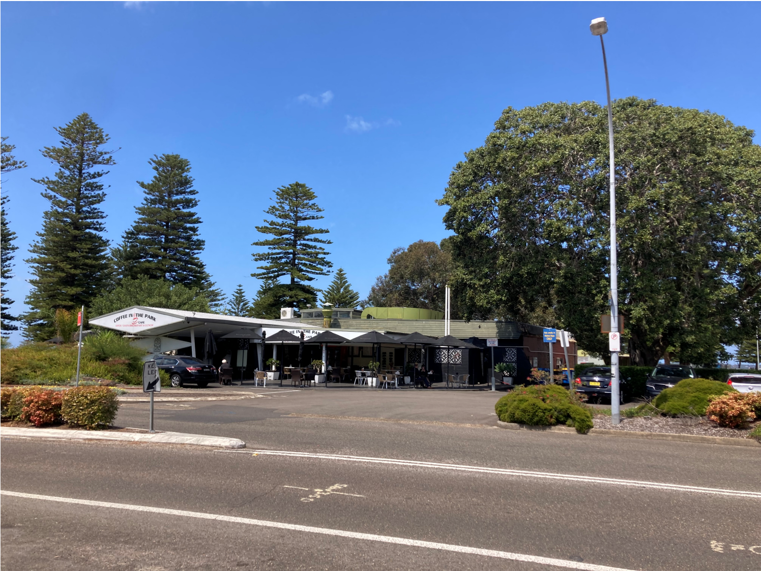
1 VIEW OF EXISTING BUILDING FROM RUSSELL AVENUE
