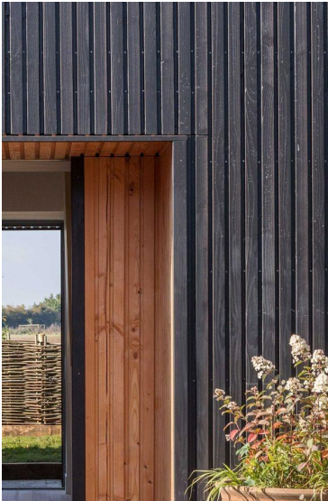
TB-01: Charred or stained dark timber cladding
