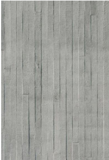
CN-01: Board formed concrete
